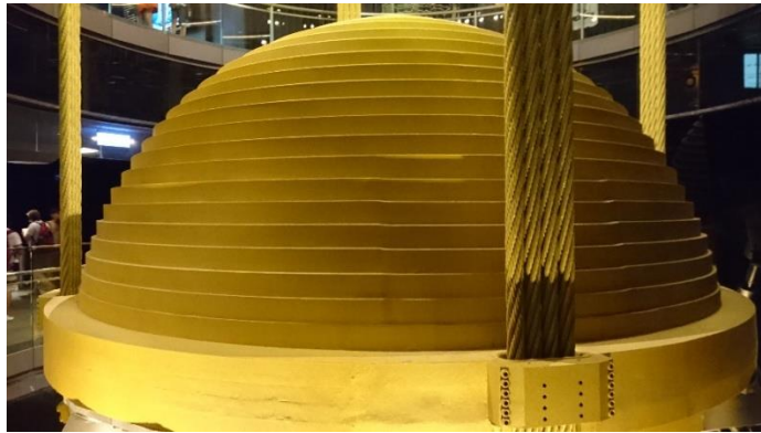
Damper ball, prevents Taipei101 shake by strong wind or Earth quakes
